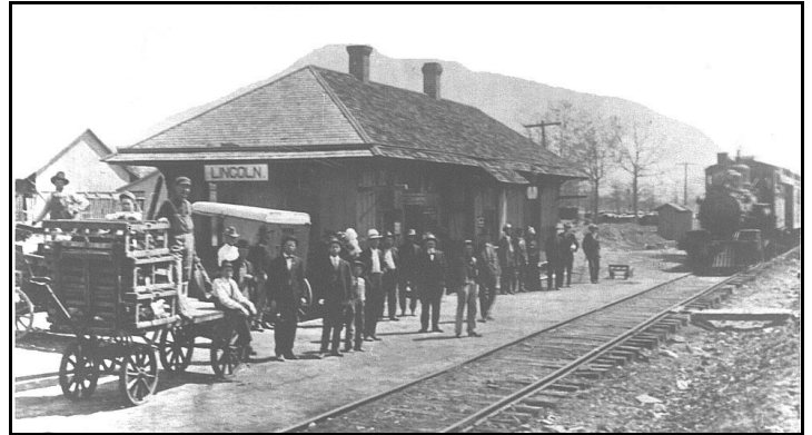
Figure 14.52: Lincoln, Arkansas Train Station.
