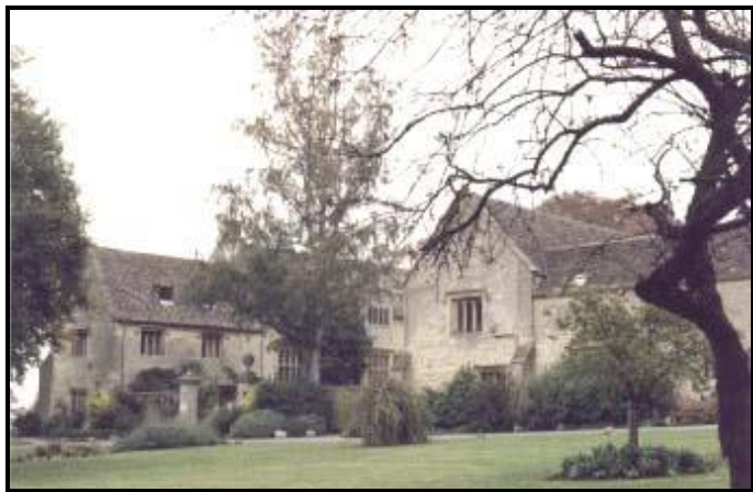
Figure 3.9: Leckhampton Manor View from without the court.
