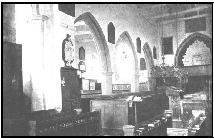
Figure 10.30: Main aisle before restoration looking toward the rear of the church.
